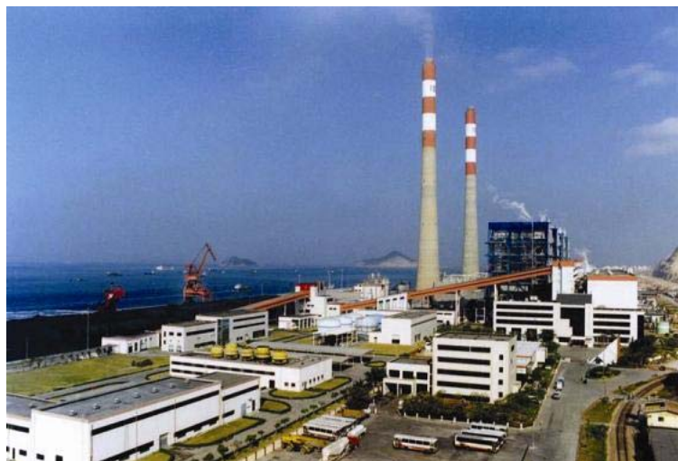
Da Gang power plant project III
